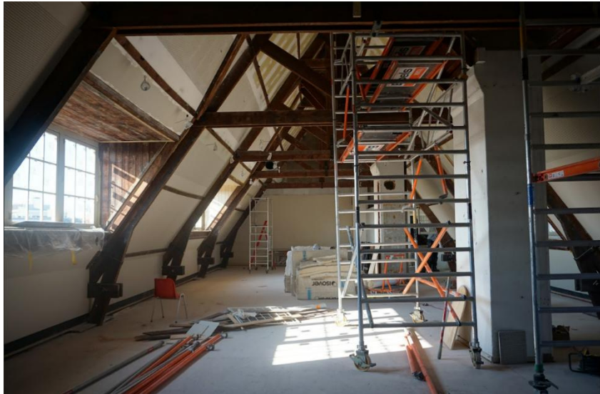
From the construction site of the Cultuur&Campus Putselaan, where different events will take place
